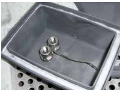
Brazing in a gas-supply box
